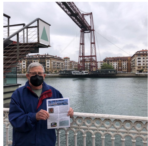
NETWORKING in Spain. Puente Colgante - Hanging bridge in Port of Bilbao, Spain. Historic UNESCO site. Iron work structure by architect who worked under Geoffrey Eiffel. Gondola-like ferry skims over the water (we road across). Can also take an elevator up and walk across. Saved travelers 40-minutes.
